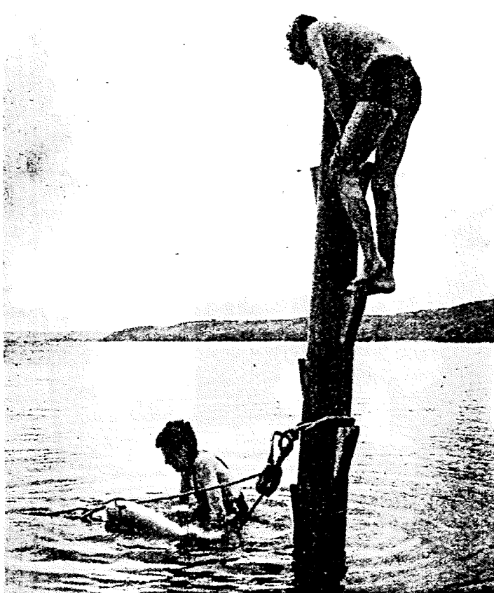
2 The Rescuing Buoy Reaches the Wreck The first shipwrecked sailor climbs in to the breeches buoy, so called because it has supports or "breeches" for the legs.
